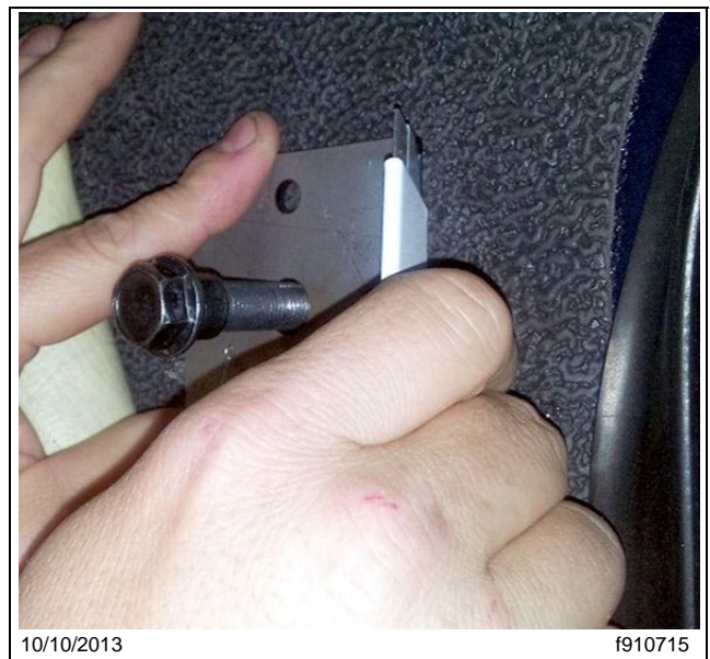
Fig. 8, Cutting for Anchor Plate
