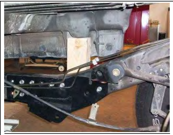
Figure 46 – Wood Block Installed at #3 Body Mount
