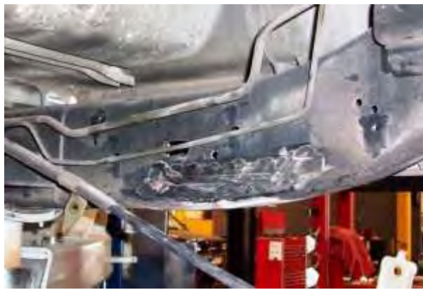
Figure 49 – Frame After Bracket Removal
