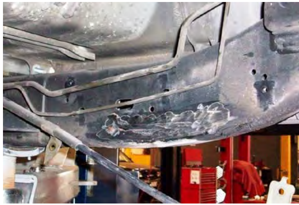
Figure 49 – Frame After Bracket Removal
