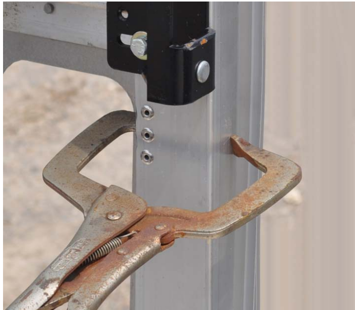
Quarter post rotation stiffener installed
