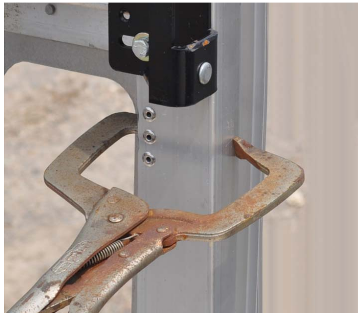
Quarter post rotation stiffener installed
