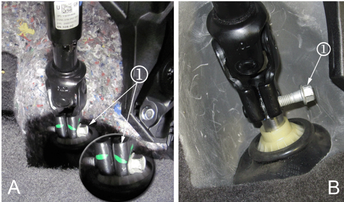
(A) Lower Intermediate Steering Shaft Bolt Fully Seated (B) Lower Intermediate Steering Shaft Bolt NOT Seated (1) Lower Intermediate Steering Shaft Bolt.
