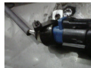
Wiring properly placed and secured with a zip tie.
