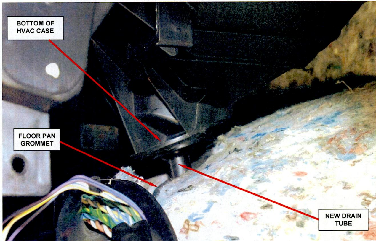
Figure 5 – New Drain Tube Installed
