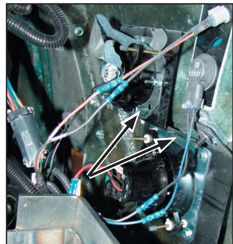
Figure 6 - Headlights and bracket assembled inside of front cap
