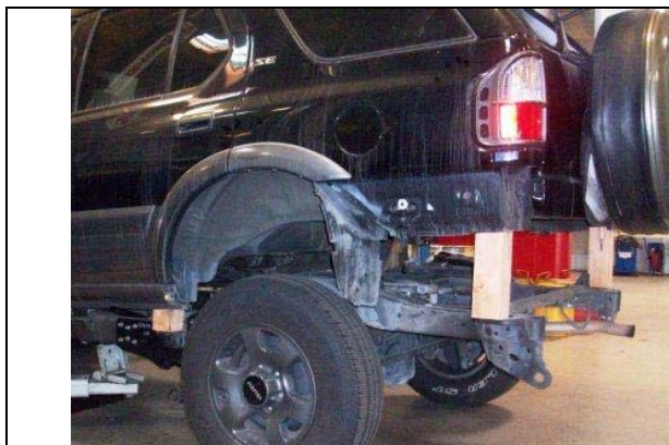
Figure 38 Wood block installed at #5 body mount
