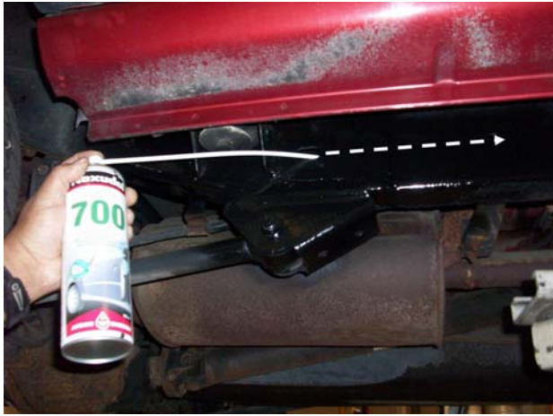
Figure 10 - Frame Hole toward front 300mm
