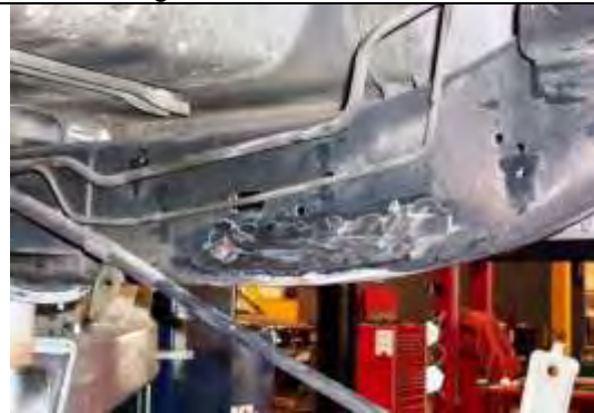
Figure 42 Frame after bracket removal
