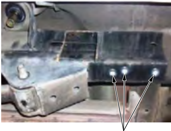
PASSENGER-SIDE POP NUTS INSTALLED
