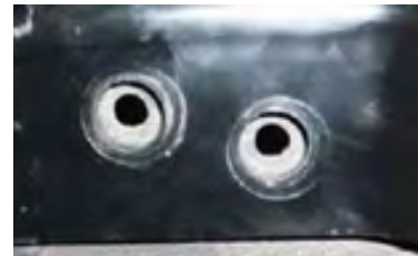
DRILLED PILOT HOLES
