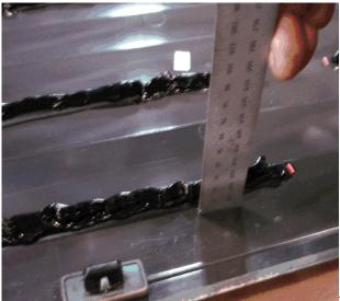
25. Ensure that the six beads of Dow Urethane Adhesive U-418 (or equivalent glass-bonding urethane adhesive) measure a **minimum** of 8 mm (5/16 in) base x 14 mm (9/16 in) height.
