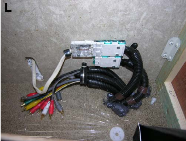
Open Molex Connector Assembly (Go to Step 3-D)
