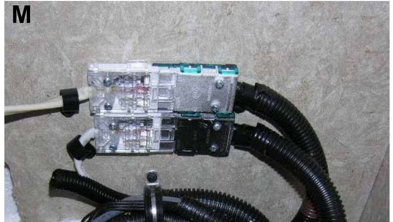
Installation Complete (No Action Needed)
