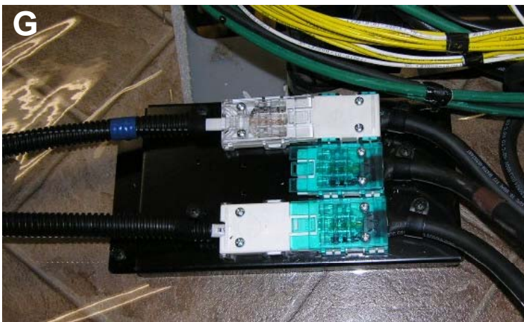
Open Molex Connector Assembly (Go to Step 2-D)
