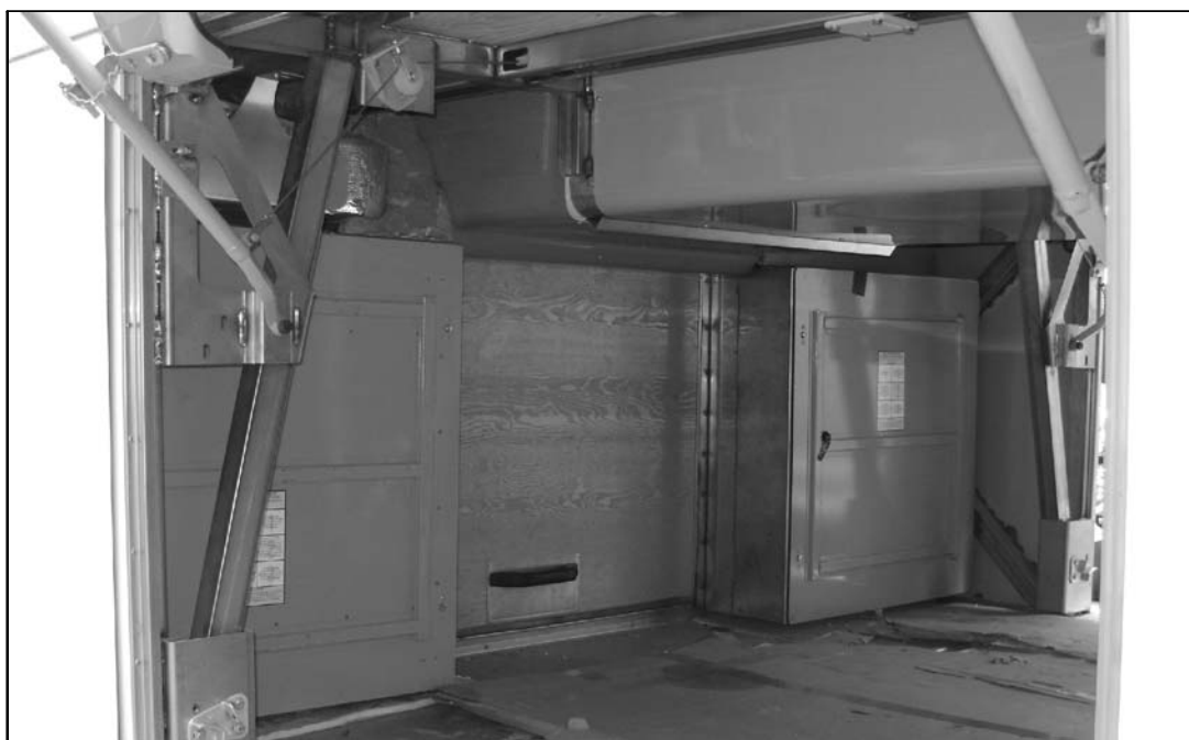
Figure 37. #3 baggage bay compartment.
