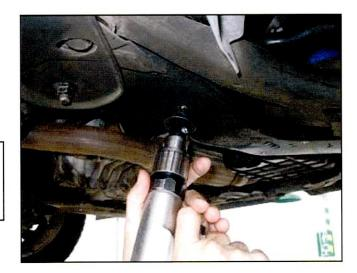
5. Debur the holes on both sides in several areas around the edges of the 40 mm hole so that an accurate judgment of the subframe material thickness can be made.
