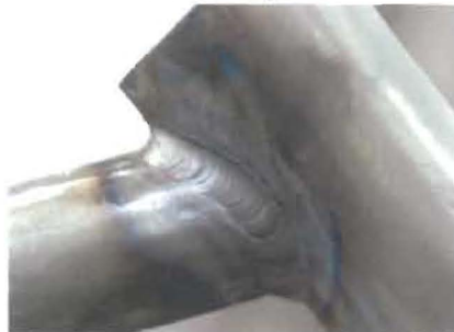
View showing the completion of the 3 rd and final weld pass
