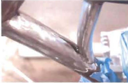
The grinder might not be able to reach all the areas for paint/powder removal
