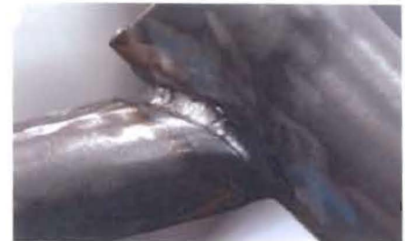
View of root pass completed
