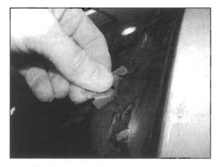
← Using a razor blade, carefully scrape away any old adhesive and primer residue
