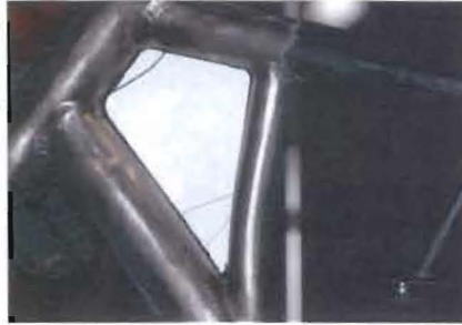
Poster board template trimmed to fit in the frame opening.
