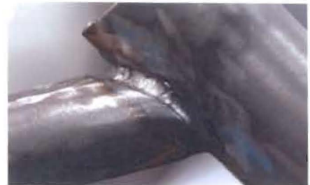
View of root pass completed
