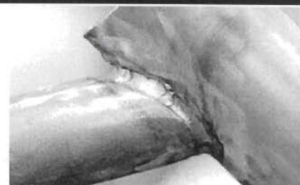
View of root pass completed
