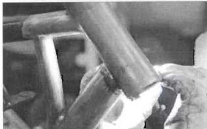
Using TIG process and 3/32" ER70 rod weld a second pass
