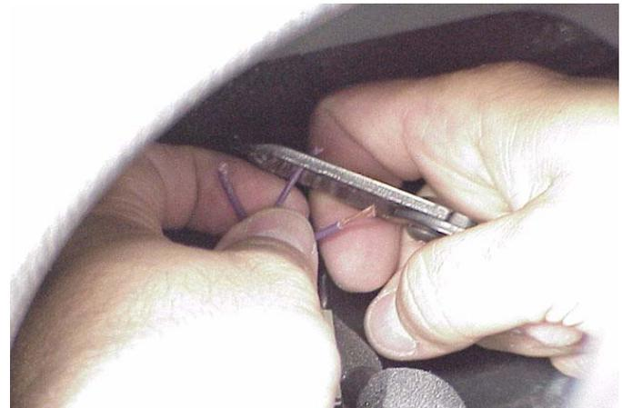
10. Insert the twisted wire end fully into the specified crimp connector. The exposed copper wire should be completely inserted in the metal barrel of the crimp connector. The wire insulation should be inside of the clear area of the connector touching the barrel.
