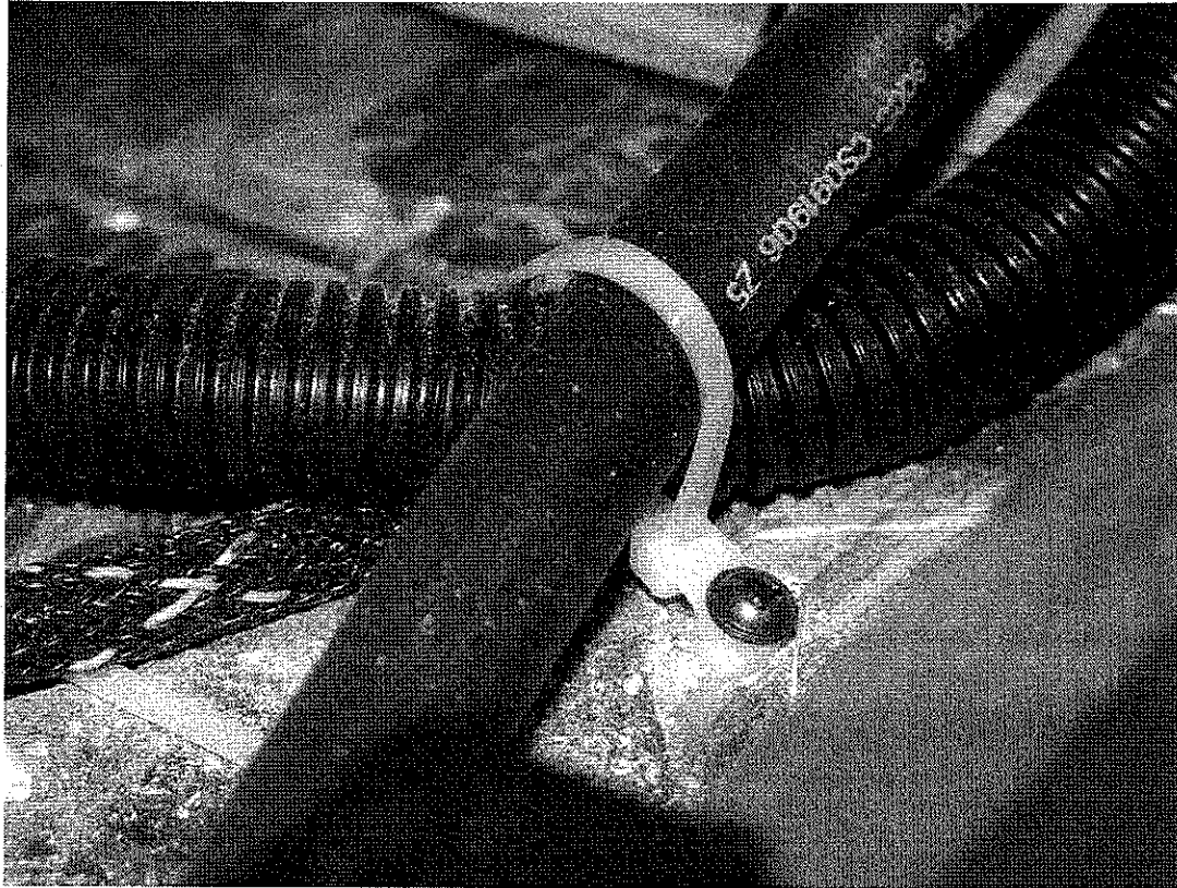
Figure 2: Anchoring the Cable Tie to the Sub Floor
