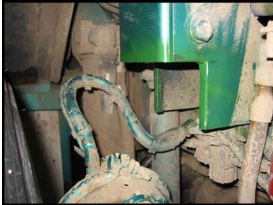
Figure 5; Hood support “after” repairs
