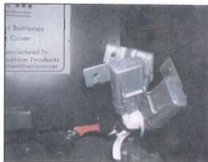
Figure 3 In-line fuses need to be located off the floor of the compartment.
