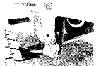
Weld reinforcing plate to this side only on front and rear hangers
