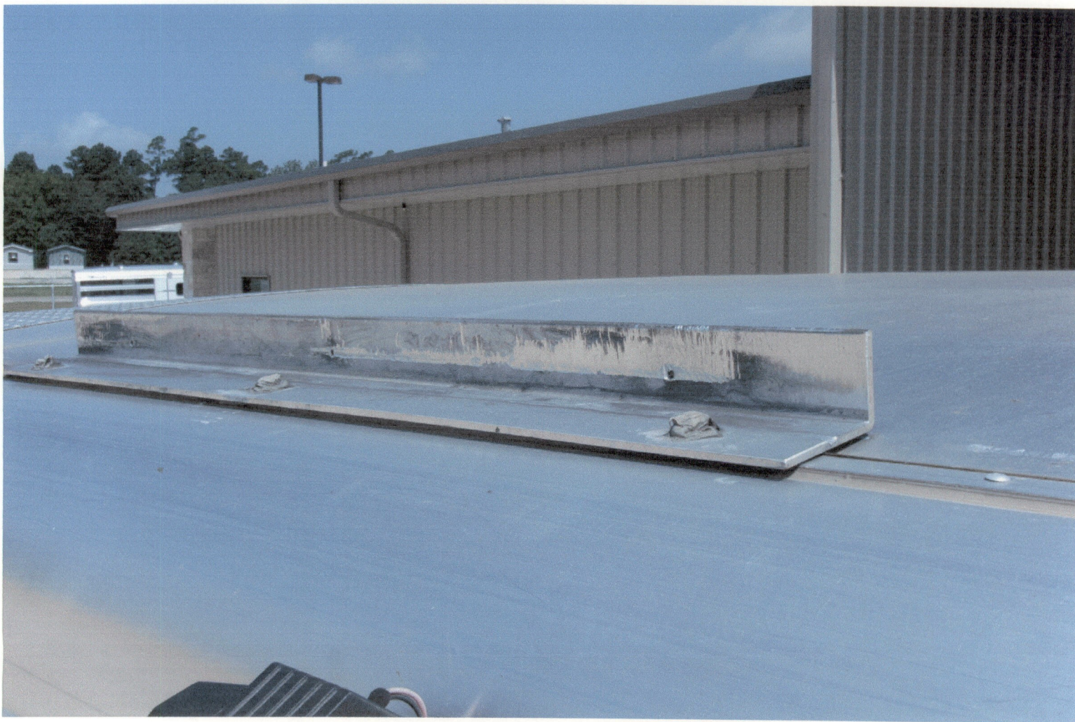
Photo of Haypod mounting bracket
