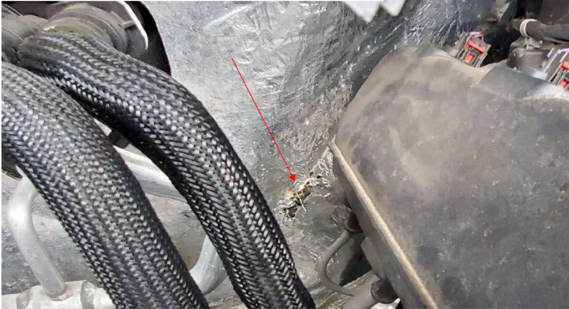
5A. Fire wall insulation damaged. Passenger side.
