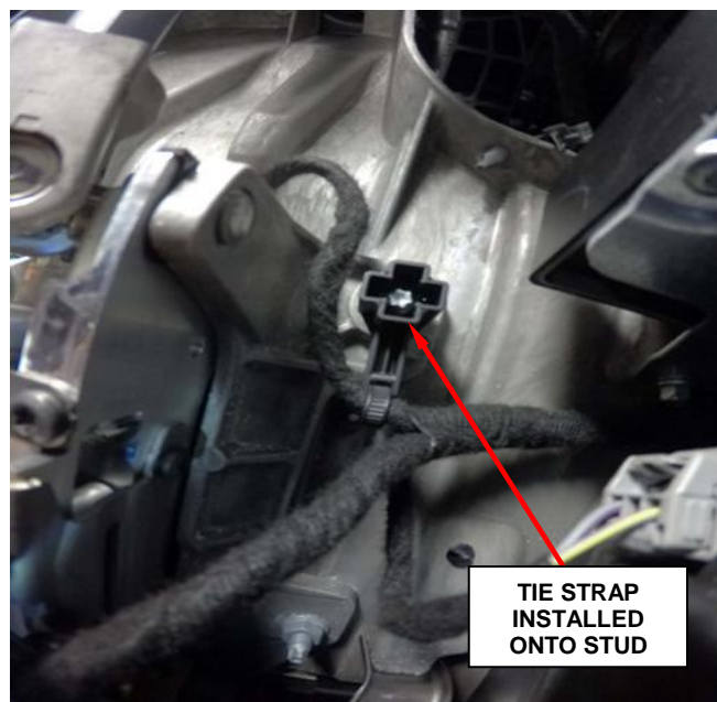
Figure 10 – Tie Strap Installed
