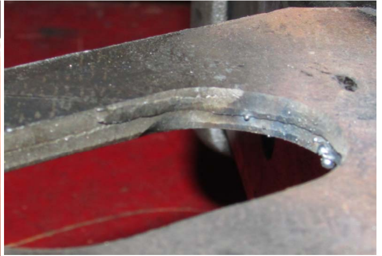
Safety Chain Attachment - Deformation
