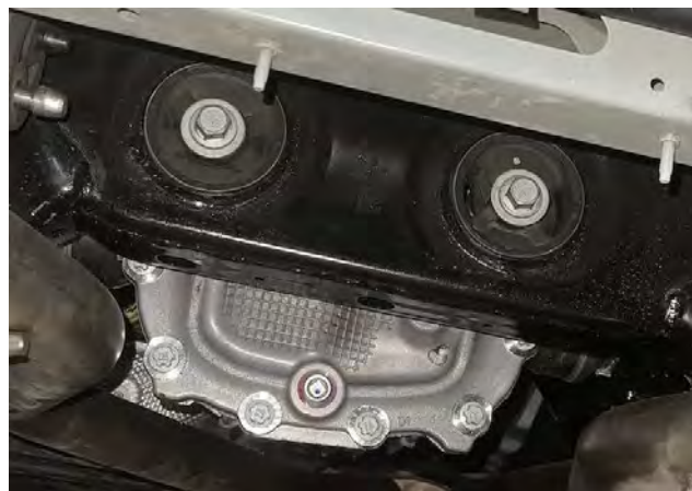
Fig. 2 – Close Up of Two Rear Axle Mounting Bolts in Fig. 1, as
