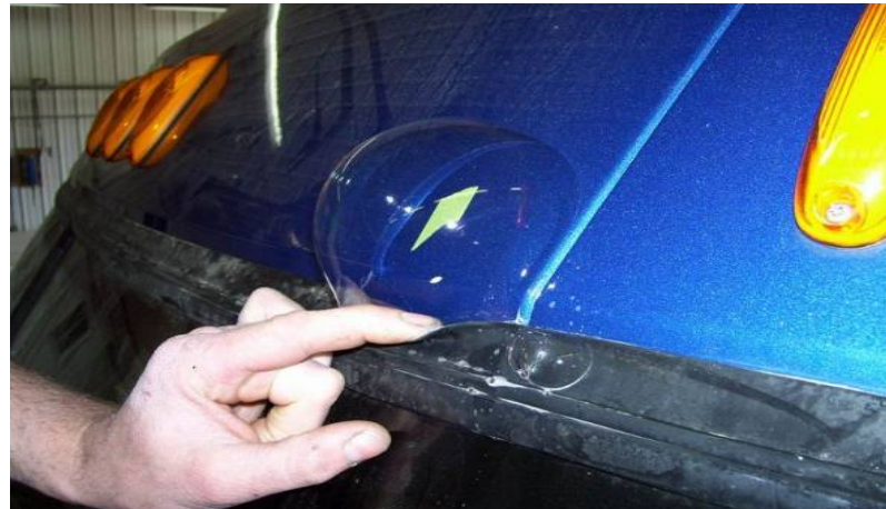
Likely leak between windshield seal and cab
