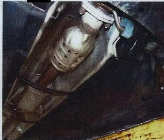
81. View of the exhaust protector.
