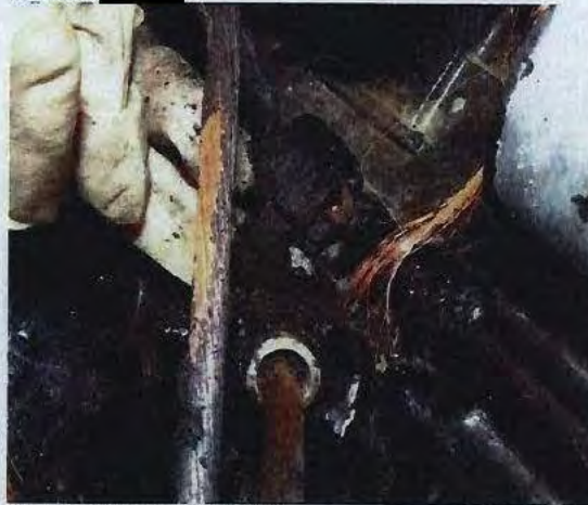
35. View of the starter cable connection.
