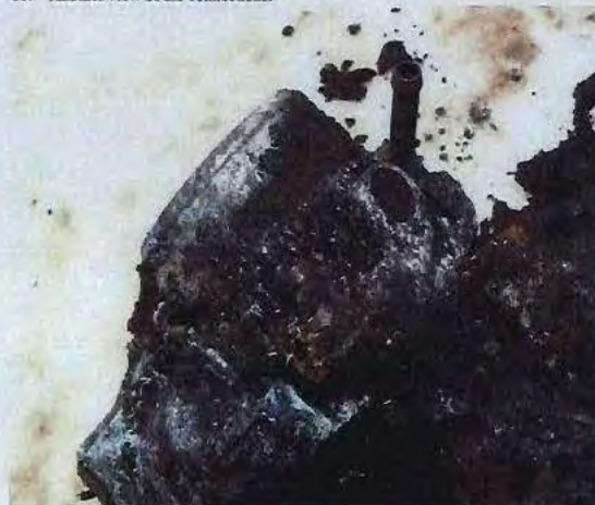
10. Another view of the connections.
