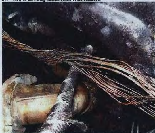
54. View of the wiring harness center of the bulkhead.
