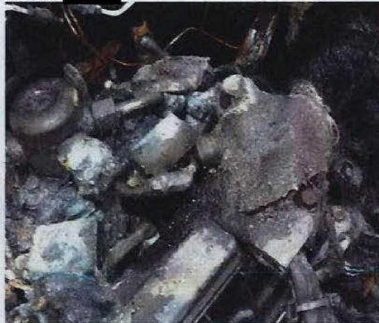
67. View of the fuel line connection.
