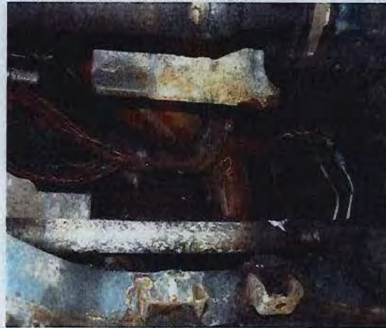
82. View of the bottom of the exhaust at the bulkhead.
