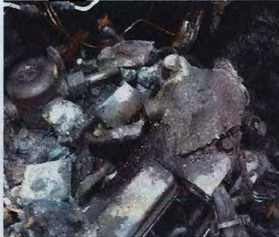
67. View of the fuel line connection.
