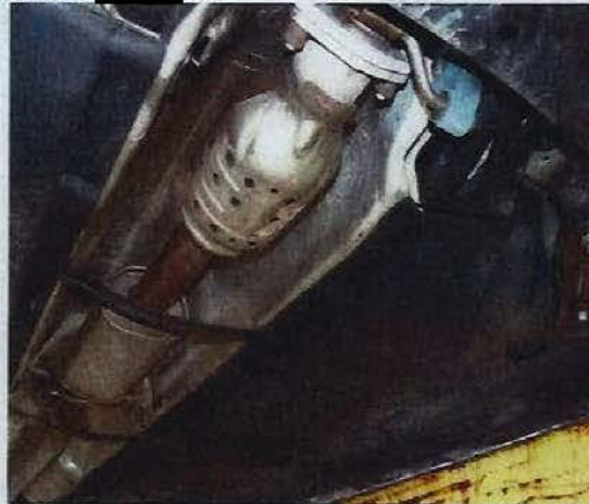
81. View of the exhaust protector.
