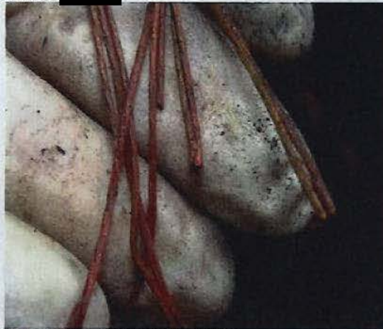
39. View of electrical activity to said branch wiring.
