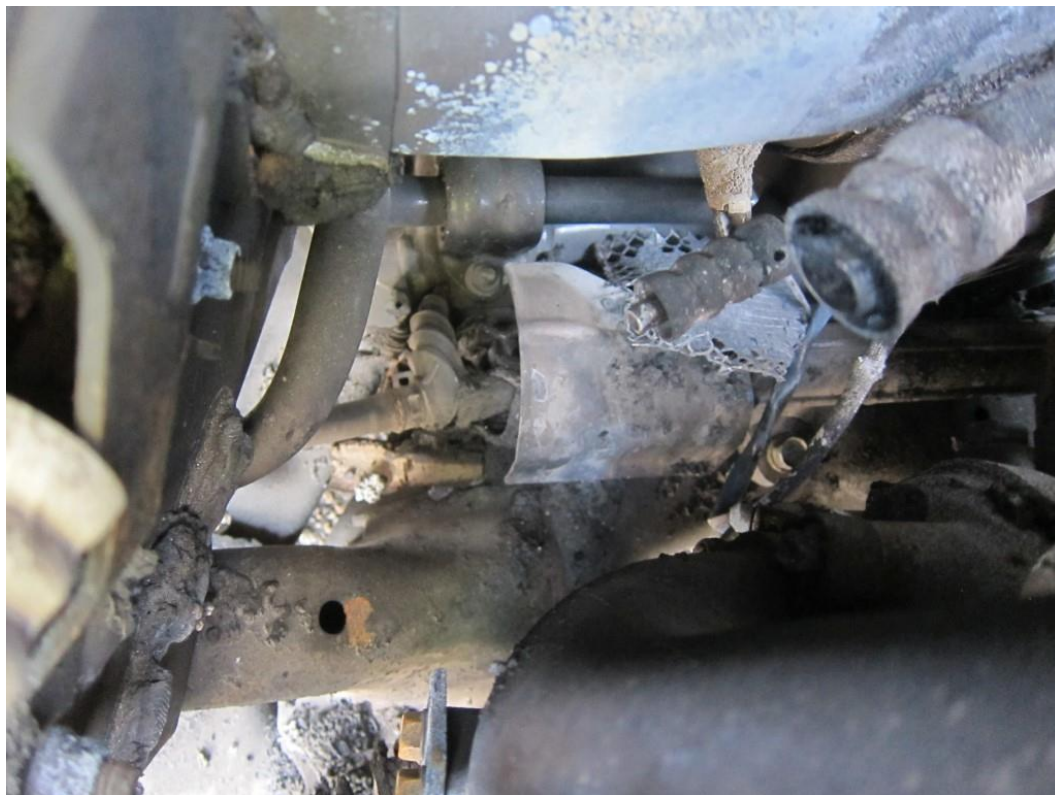
Photograph 15. Right side of the steering rack.
