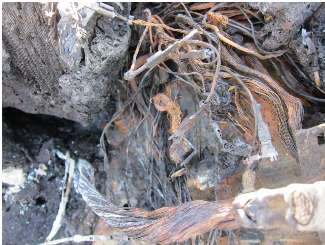
Photograph 23. Close-up of short-circuit area of the engine compartment fuse box.
