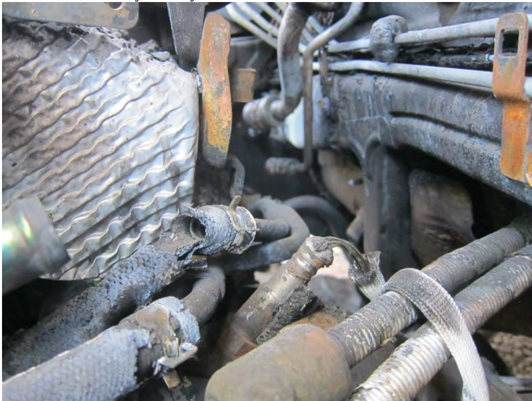
Photograph 12. Fire damage to the rear of the engine and turbocharger area.
