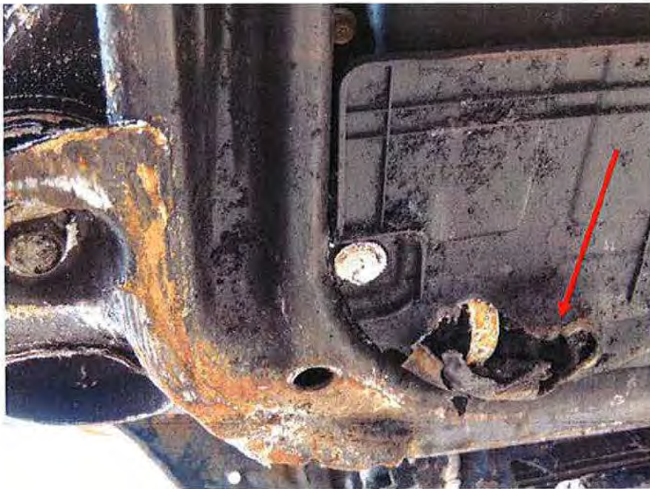
12 The red arrow depicts a area that should be removed to identify any concerns of electrical activity
