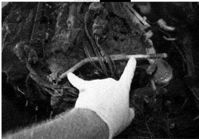
Photo No. 11: View of metal fuel line crossing over engine
