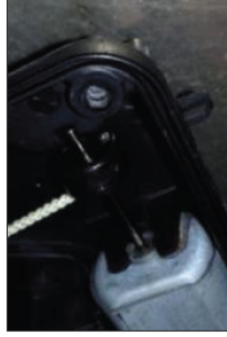
After KV operation at test box with open circuit cord fully unwound → OK
