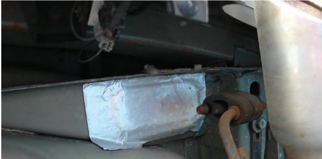
Figure 14. Mastic patch applied to underside of Explorer as part of CSP 17N03 repairs.
