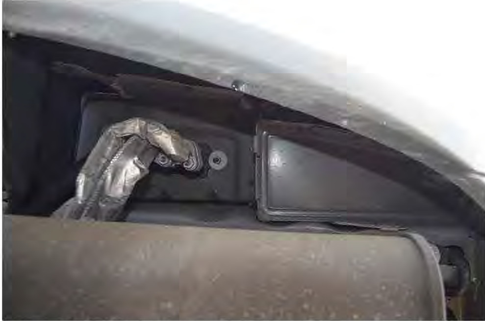
Figure 41. 2015 Ford Explorer Limited 9474 lack of underbody sealing.
