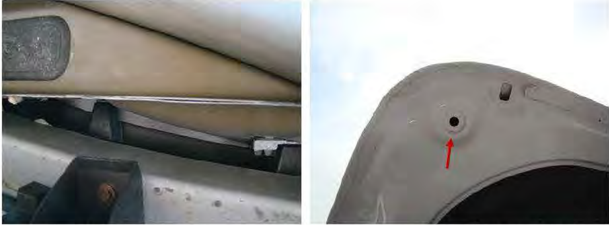
Figure 8. Lack of underbody seam sealant and liftgate valves on the [redacted] 2013 Ford Explorer 1363. Note the missing liftgate bumper in the right photograph.
