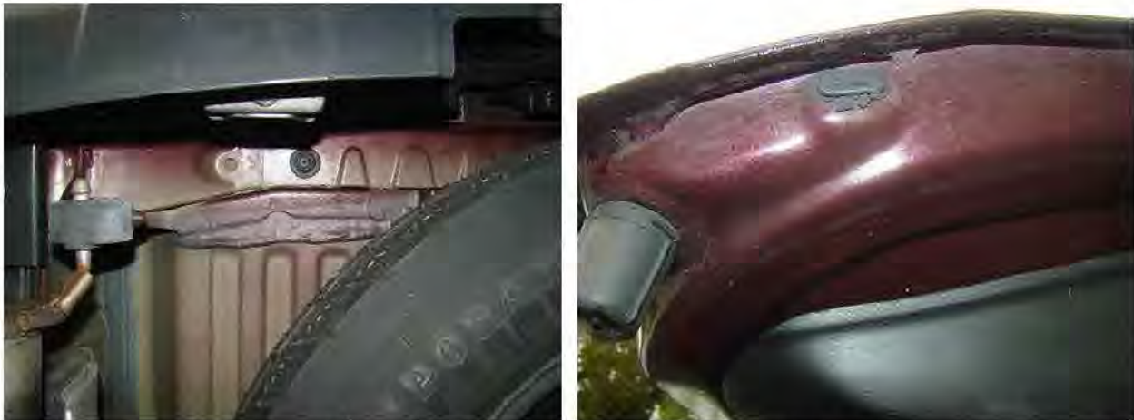
Figure 38. 2011 Honda Pilot [REDACTED]. Intermittent underbody sealant at left. Plugged drain holes on the left and right sides at the latch end of the liftgate.
