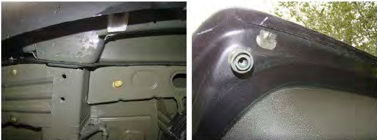
Figure 32. 2016 Chevy Traverse 2347. Intermittent underbody sealant at left. Plugged drain holes on the left, middle, and right sides at the latch end of the liftgate (top of photo).
