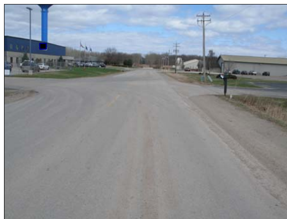
Figure 2: Freightliner's eastbound approach to the driveway (on right) and area of explosion
