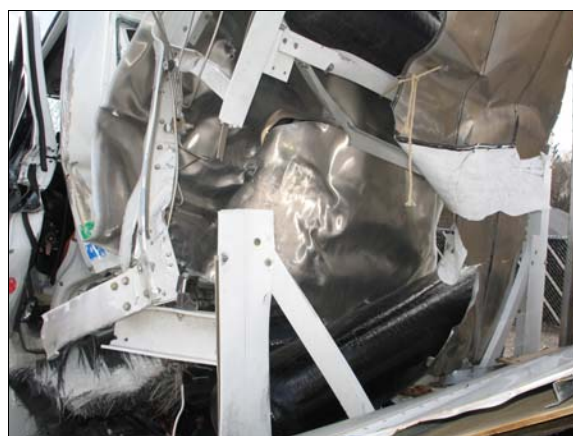
Figure 12: Exterior view of intrusion of back wall of Freightliner's cab
