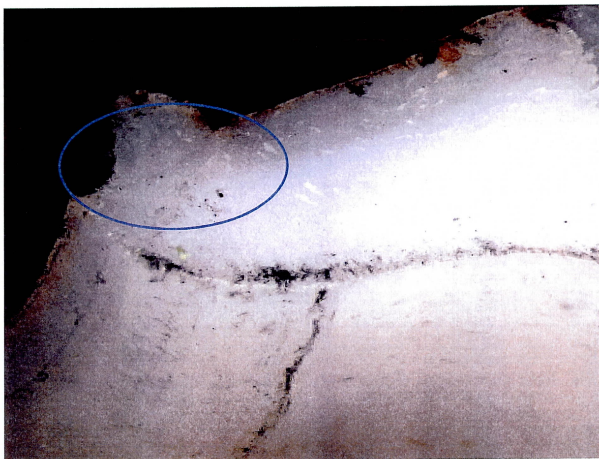
Cracks at insert groove.
