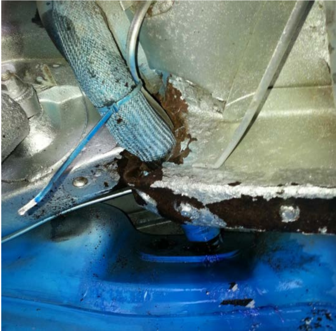
Figure 12 - Test #3 Significant rust causes collapse at relief tunnel in rail where fuel hoses pass through
