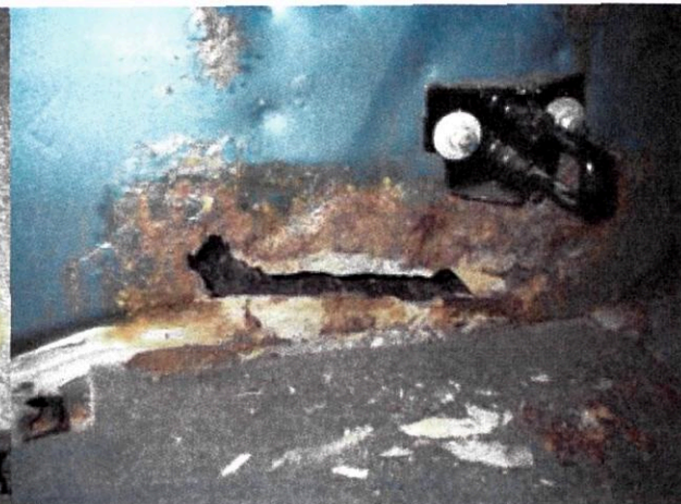
Figure 4 Increased Corrosion of Anchor Loop
