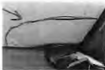
RT LOWER CORNER GATE BENT L4
