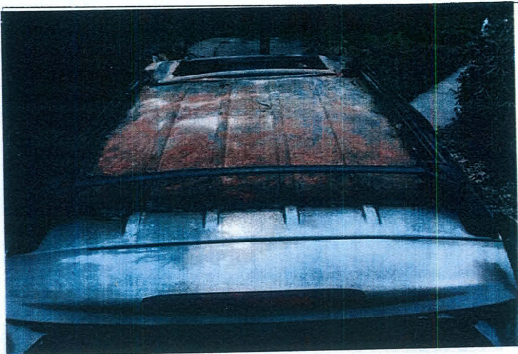
PASSENGER COMPARTMENT (PC) ROOF FROM THE REAR
