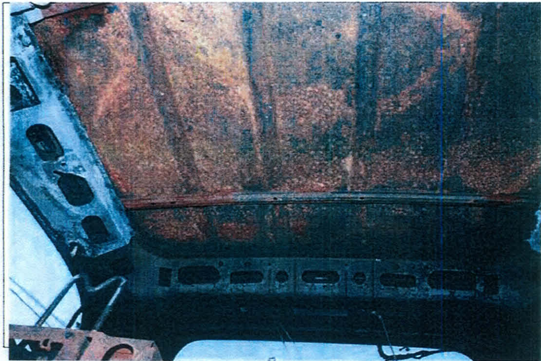
CEILING ABOVE REAR PC STORAGE
