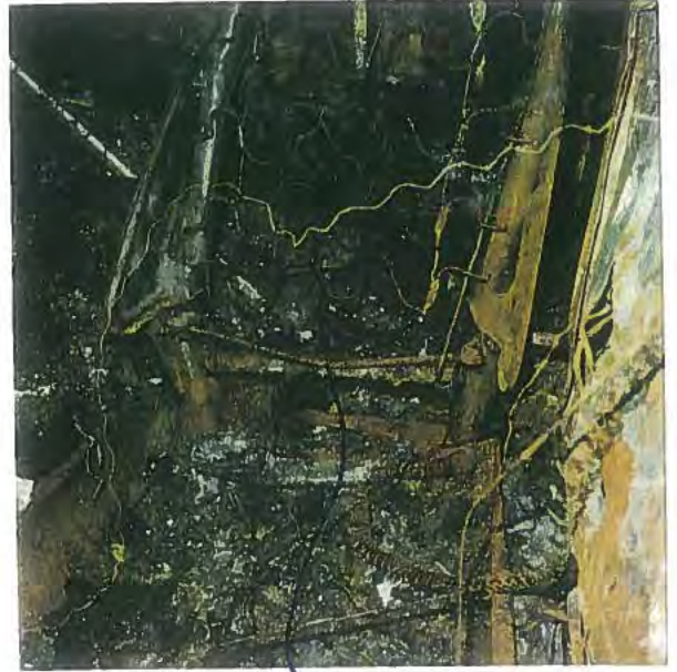
ADJUSTER ROD BUCKLED IN COMPRESSION
