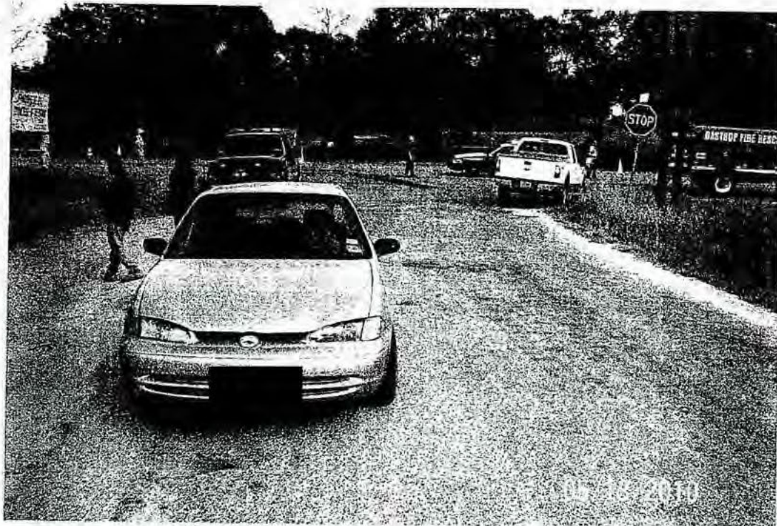
5. Travis Road facing south, looking towards SH 21
